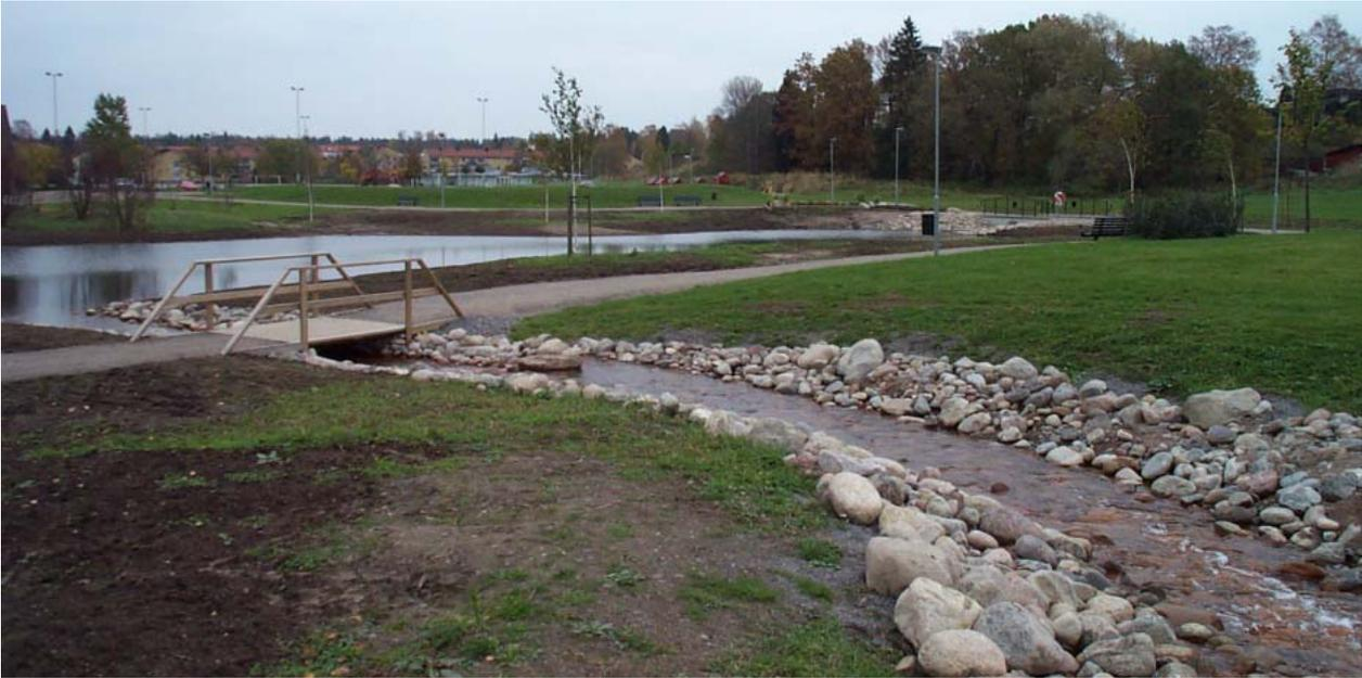
**Figure 5** A wet pond facility in Fornudden, Tyresö. A result of the first watershed management plan.
